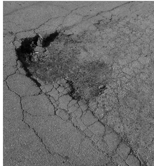
Figure 2 : Stripping in asphalt pavement due to lack of bond b/w asphalt and aggregate
